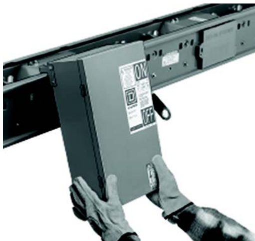
Figure 109: Plug-In Device Mounting
